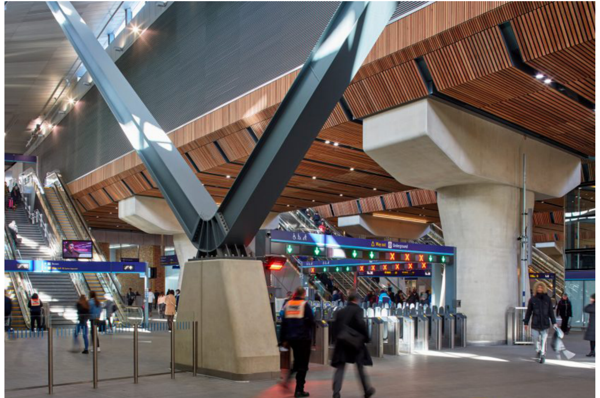
Fig. 2 London Bridge Station
