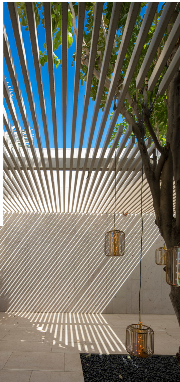
Fig. 5 House built on a cross plan - slatted ceiling
